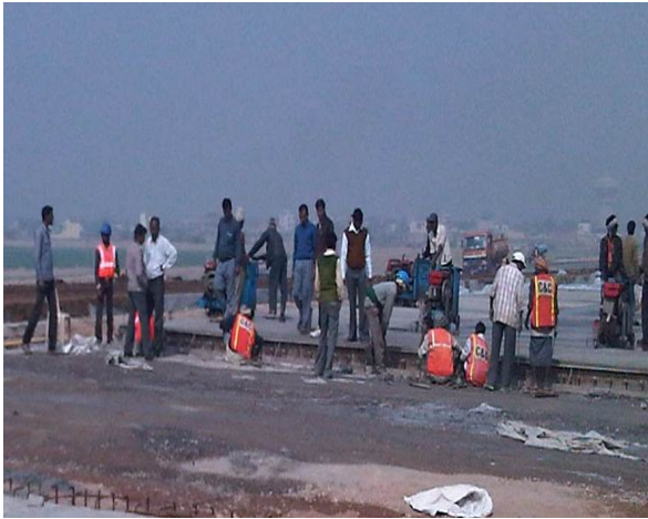
Yamuna Expressway construction site
